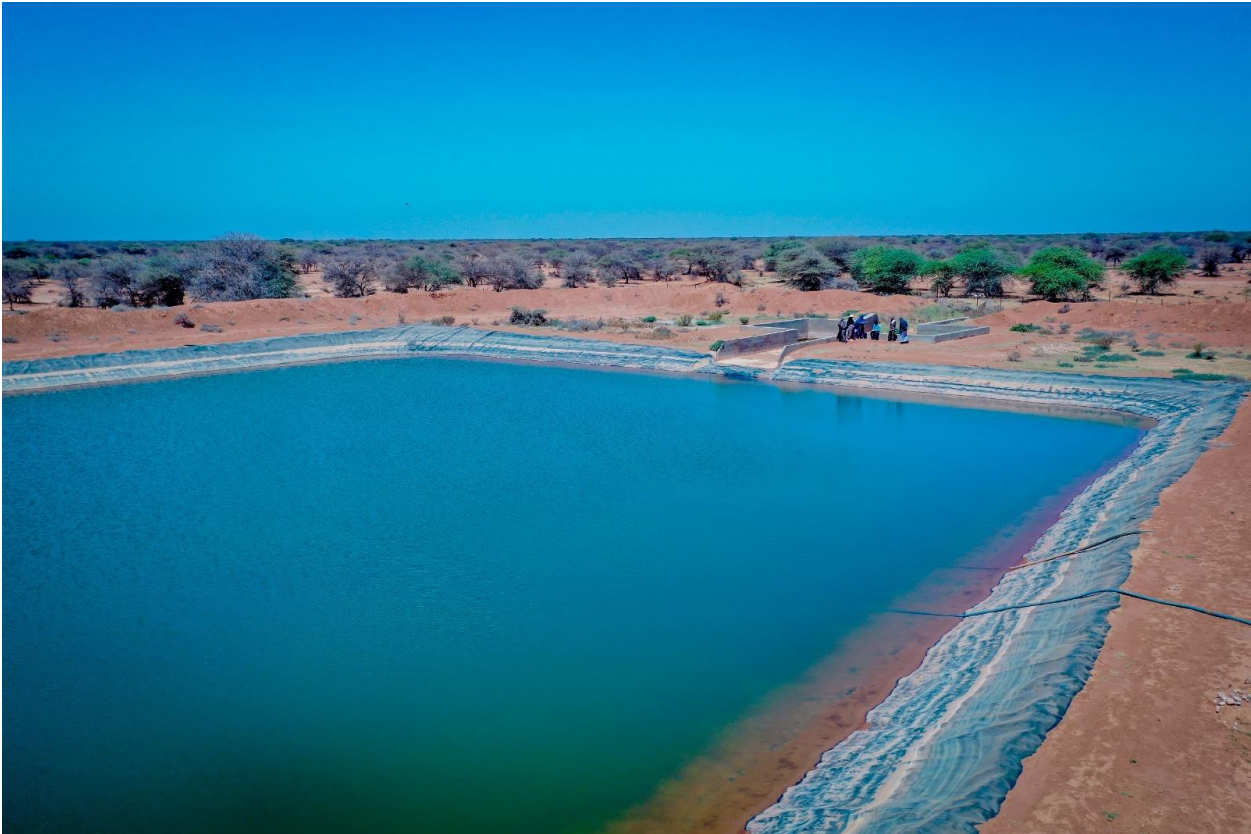
Figure 36: The haffir dam near the project site
