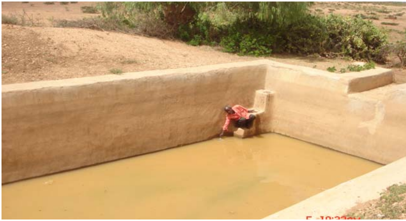
Figure 4.1 Rectangular berkad with concrete wall
