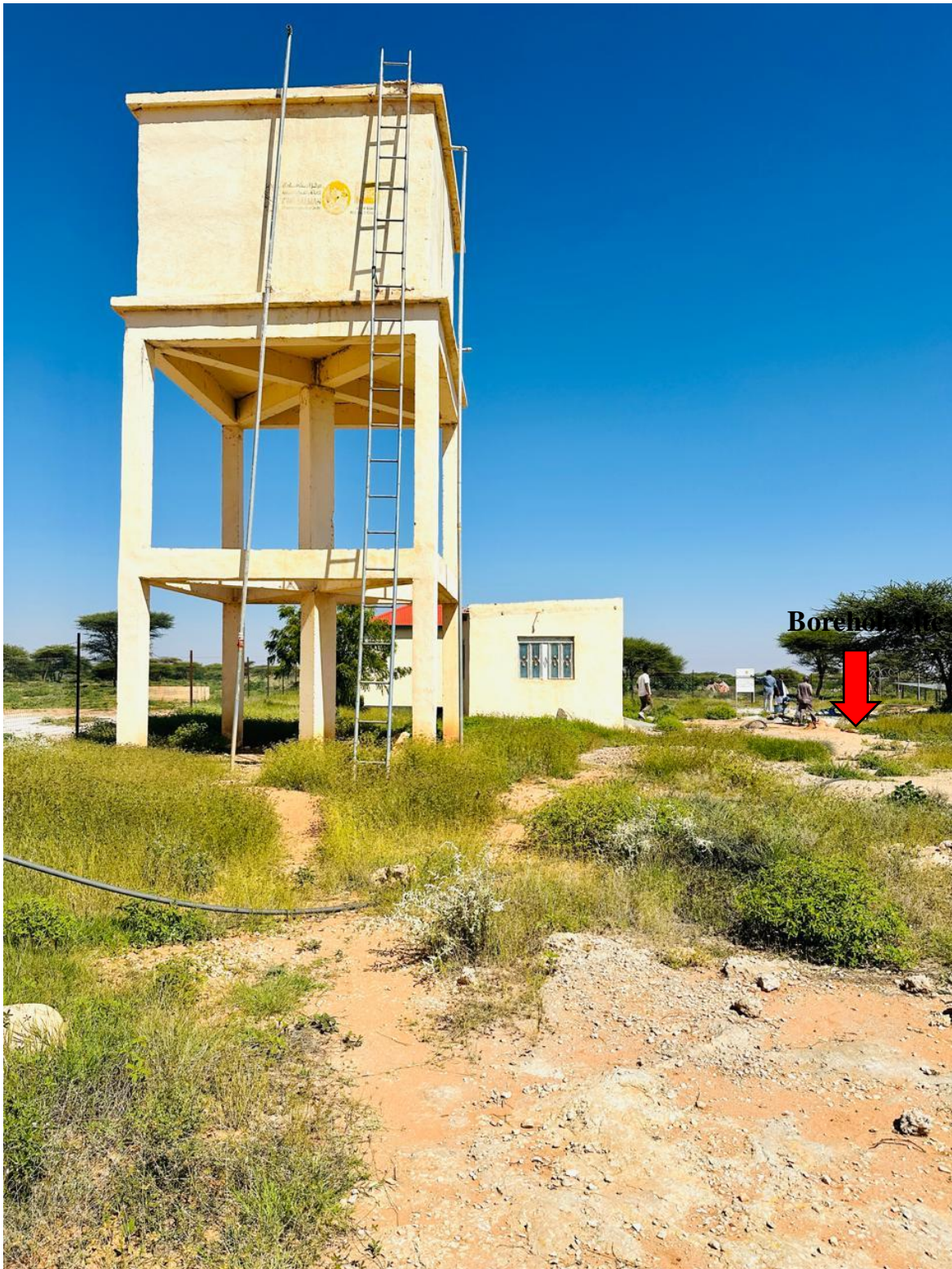
Figure 2: Guryosamo Borehole Site, Reservoir and Generator room
